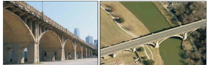
Figure 4 – Houston Street Viaduct (Dallas) and N. Main Street Bridge (Fort Worth)
