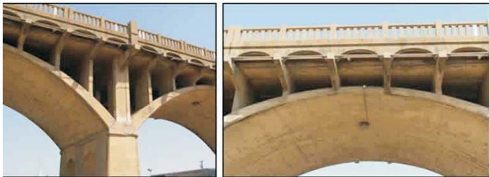
Figure 3 – Structural System of the Congress Avenue Bridge
