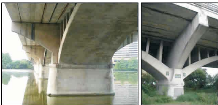
Figure 7 – Pier Cantilever Extensions
