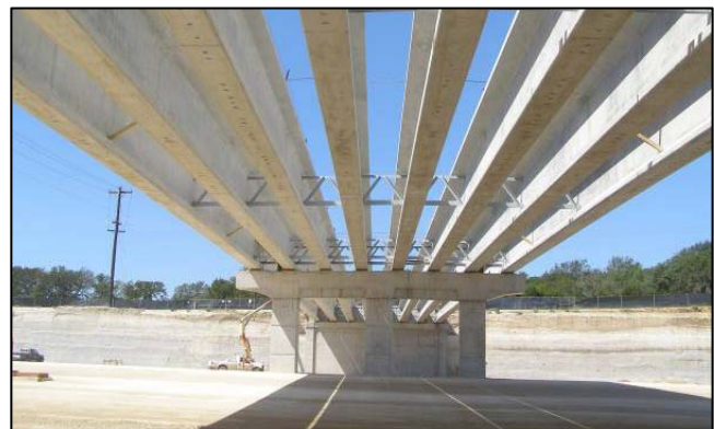
FIGURE 10 – PARK STREET BRACING
