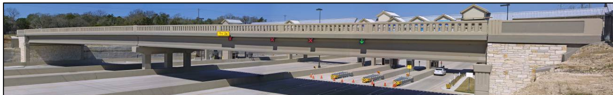
FIGURE 8 – PARK STREET BRIDGE
