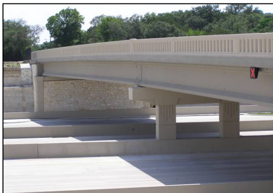
FIGURE 9 – PARK STREET BRIDGE
